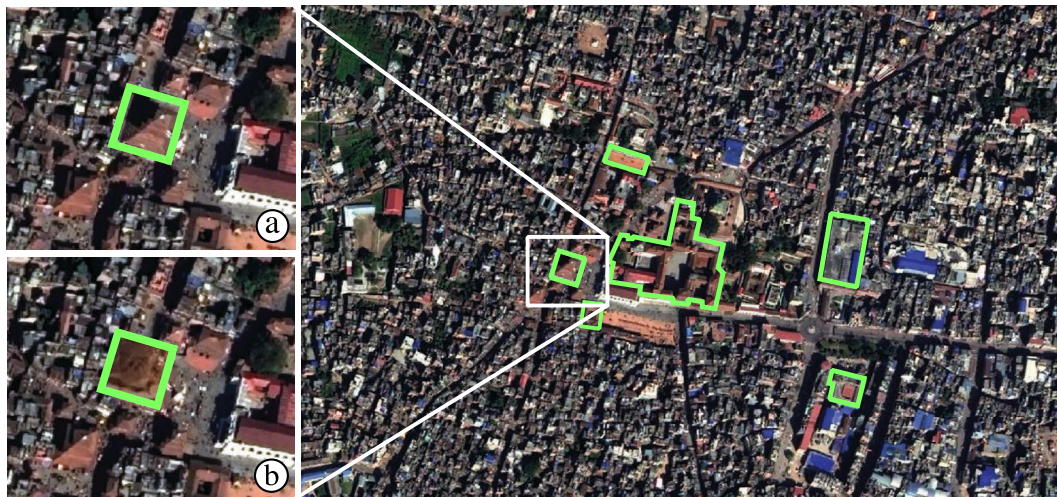
Figure 6. Nepal earthquake, 2015. Compositing vector objects to quickly identify buildings of interest and make a preliminary damage assessment. (a) Close-up on a building, showing imagery captured before the disaster. (b) Compositing post-event imagery inside these buildings only.
