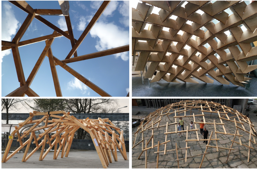
Figure 1: Physical RF-structures designed and fabricated by architects: a simple roof structure (top-left), a design by Michael Clarke (top-right), a design from Spiro-ETH (bottom-left), and a design from Wan Shu and Kengo Kuma (bottom-right).
