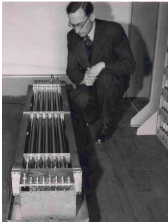
Figure 8: Wilkes and Mercury Delay Lines
