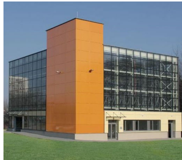
Fig. 1. A view of the Automated Transportation Center in Ostrava
