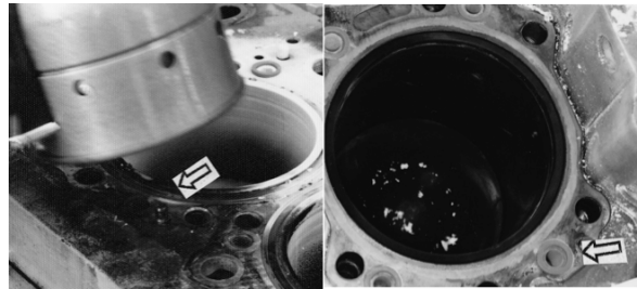
Fig. 11. Detected Coolant Leakage on Engine Bench Test Right: Detected Coolant (arrow mark) Left: Leaked Seal (arrow mark) (S. Ohkawa et al. 1993 [3])
