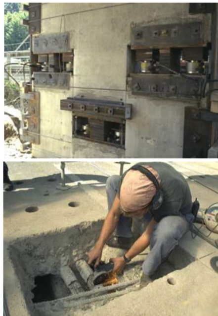
Figure 2. Chronological overview of applied damage scenarios (left), settlement system used for damage scenarios 3 - 6 (right top) and cutting of tendons for scenarios 15 - 17 (right bottom). [12].
