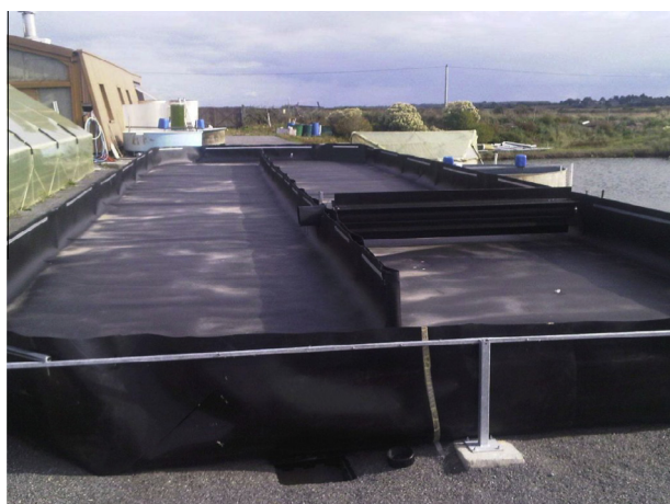
Fig. 2. Alpha Biotech raceways for algal biomass production, Gu erande, France.
