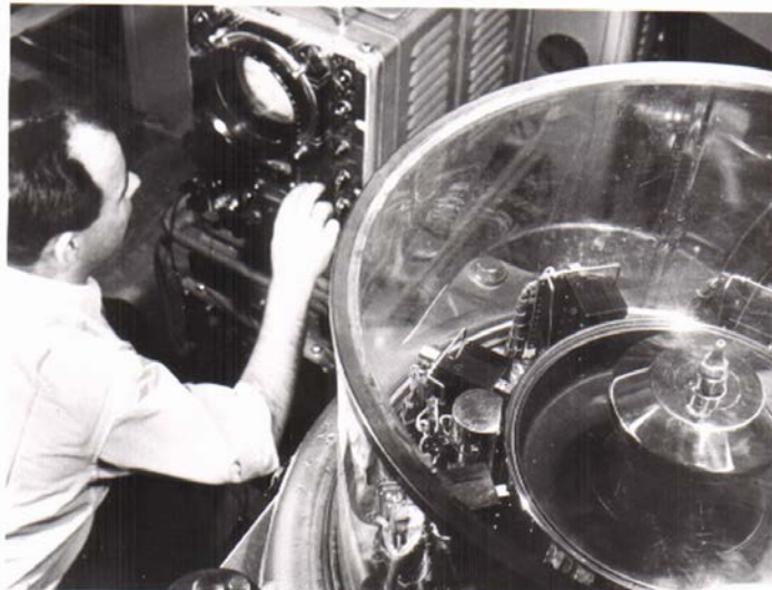
Fig. 2. Gy. Kovacs and the drum memory of the M-3
