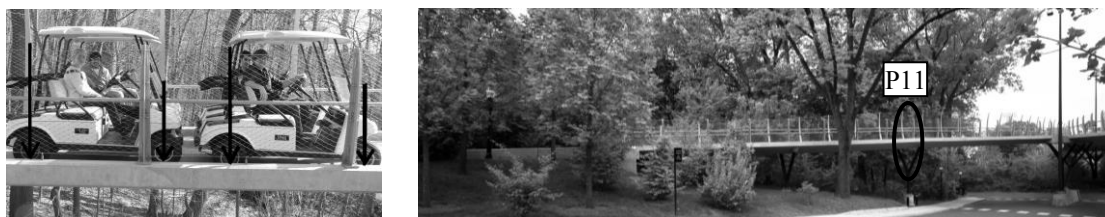
Figure 2: Left: Load test, the bridge was loaded with four golf carts. Right: Location P11 is above a support.
