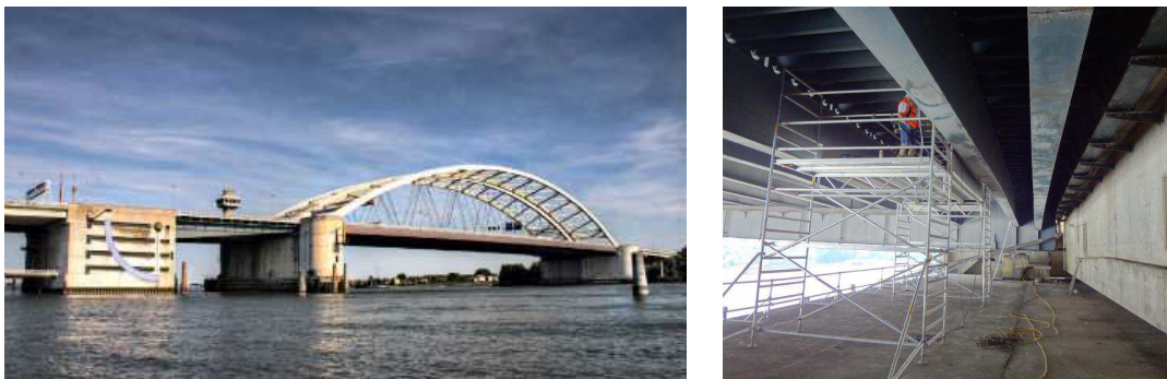
Figure 9. Van-Brienoord bridge in Rotterdam (left); installation of the sensors (right).
