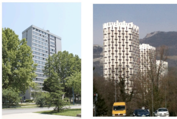
Figure 2 Description of the Buildings (left: Arpej buildings; right: Ile Verte towers)
