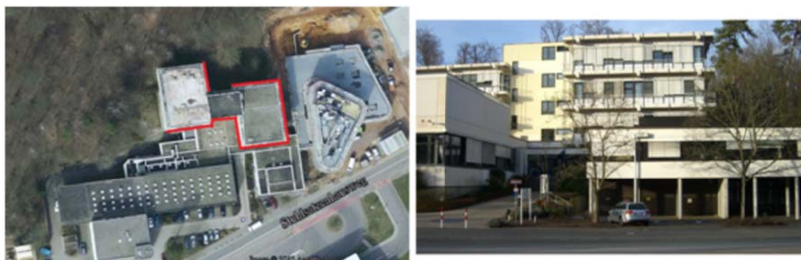
Figure 2: Left: Aerial view of Fraunhofer IZFP building with rendered line indicating inspection facade. Right: Front view of the Fraunhofer IZFP building.
