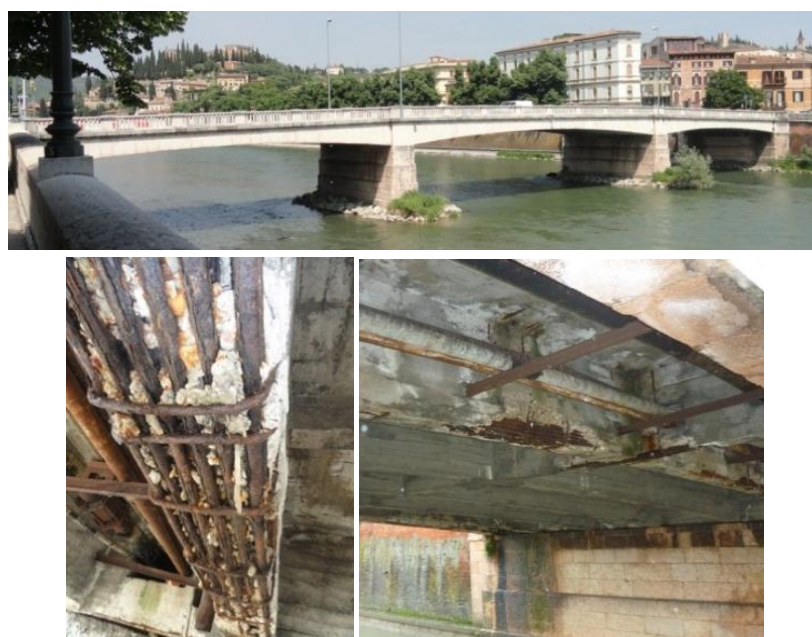
Figure 2: Ponte Nuovo del Popolo and its damaged girders.
