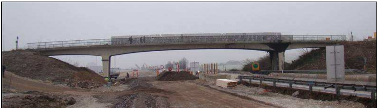
Figure 1. Bridge S101 during damage test [25].
