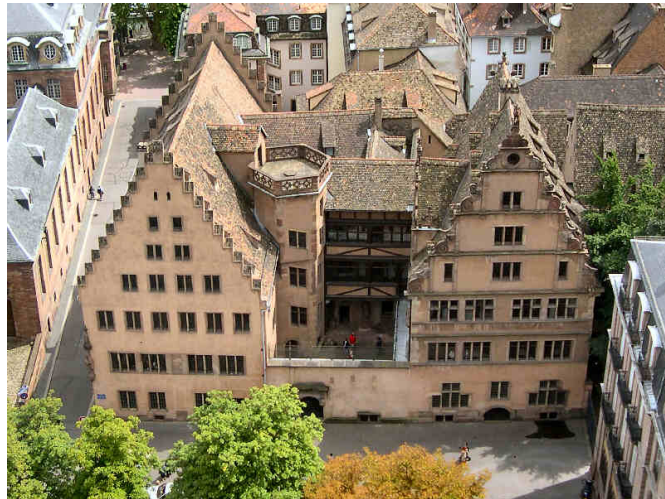
Figure 1: The Musée de l’Œuvre Notre-Dame in Strasbourg. The staircase is located within the hexagonal tower between the two buildings. (Wikipedia)
