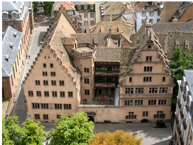
Figure 1: The Musée de l’Œuvre Notre-Dame in Strasbourg. The staircase is located within the hexagonal tower between the two buildings. (Wikipedia)
