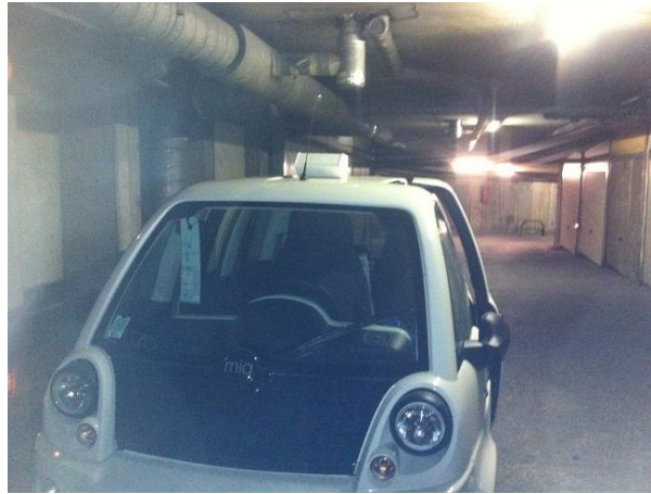
Figure 51: EV-based sensors ( equipped MIA)
